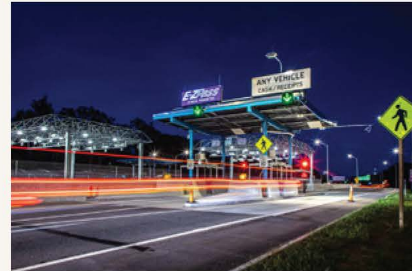
The Turnpike's first highway-speed Open Road Tolling gantry opened in 2013. Now there are six ORTs keeping traffic flowing.
