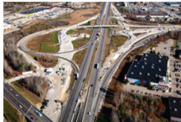
At Exit 45 a safer, more efficient diamond interchange will streamline access to and from Interstate 295, the Scarborough Connector, and Route 1.
