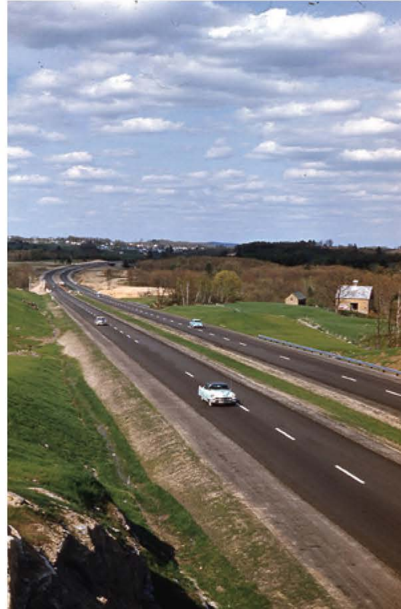
Next time you're on the Turnpike, note the long, straight stretches and gentle curves that minimize the likelihood of vehicle accidents and permit high-speed driving.
