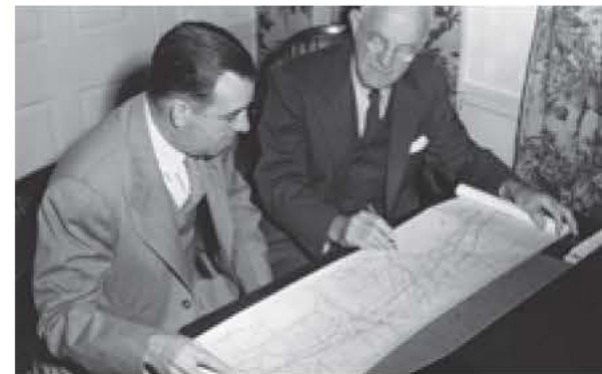
H.D. Harding, District Manager for Esso and Joe Sayward, the Turnpike Authority's first chairman review plans for the Howard Johnson's/Esso service plaza in Kennebunk.
