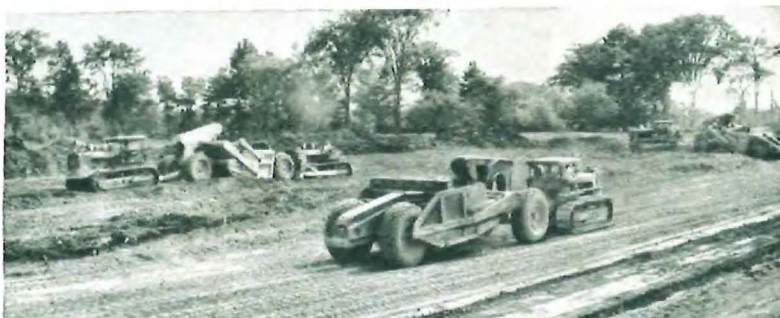
DIGGIN' IN FOR DEMATTEO. "After six weeks of rain it's mighty nice to see our TD-24s delivering 24 cubic yard payloads to help us get back on schedule" reports F. L. Kirby, superintendent for DeMatteo Construction Company, Quincy, Mass. Eight TD-24s are on the job.
