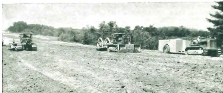
IT'S TD-24s 9 TO 5. The Savin Construction Corp., East Hartford, Conn., uses 9 INTERNATIONAL TD-24s on its 10.585 section of the Turnpike to move 2,000,000 cubic yards of earth and 90,000 cubic yards of rock. Three TD-24s shown compacting a fill near Portland.
