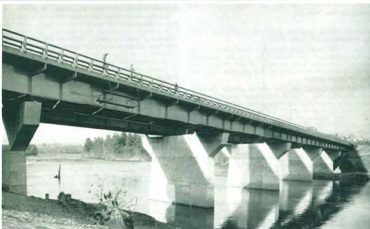
ANDROSCOGGIN RIVER BRIDGE AT LEWISTON, MAINE carrying the Augusta Extension of the Maine Turnpike 6-span continuous plate girder bridge, 845'—8" long
