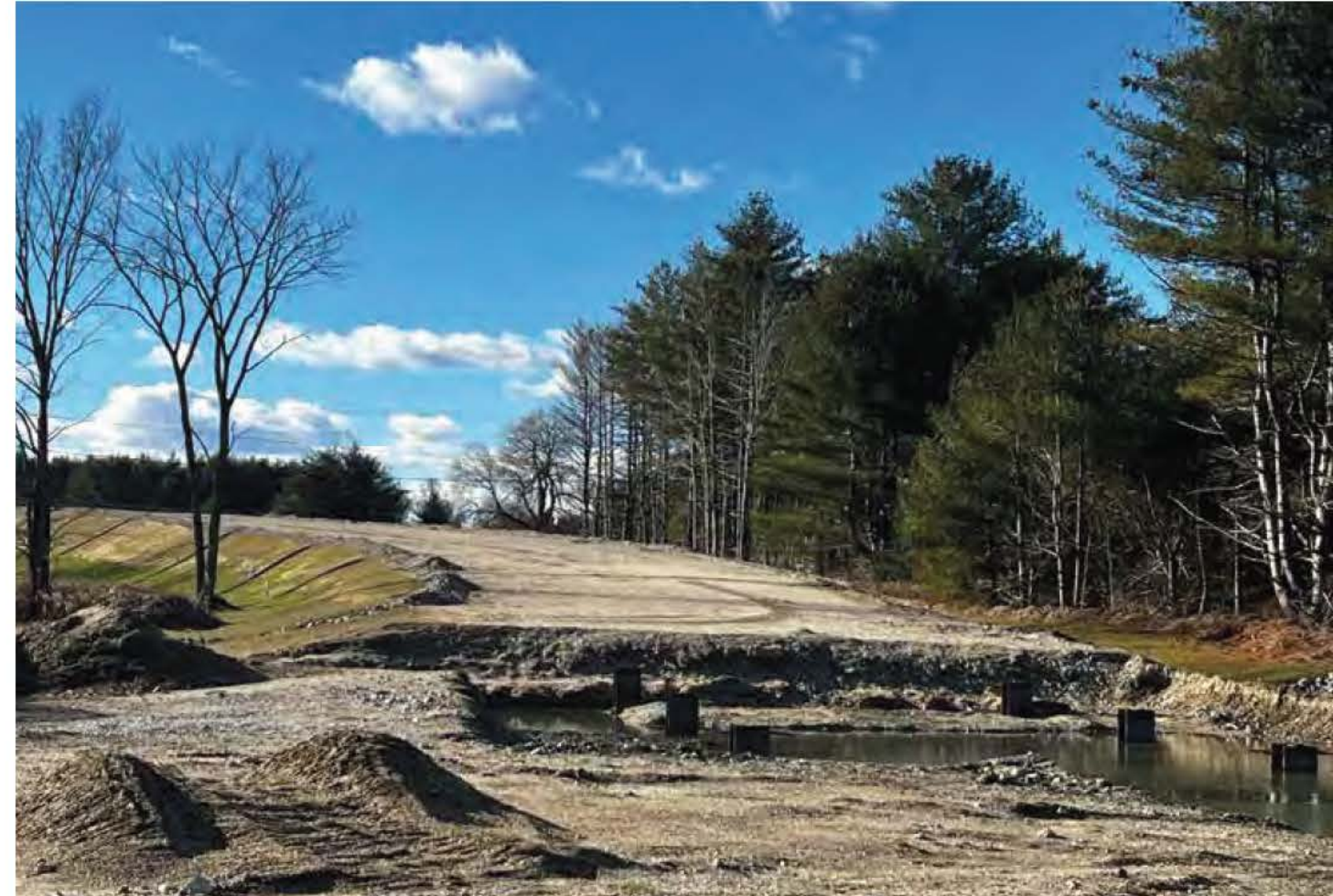
Material from the former bridge approach was reclaimed, processed, and reused as structural fill, reducing waste and supporting the new project's foundation
