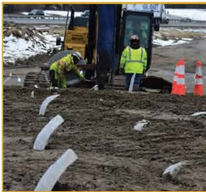
Placing wick drains
