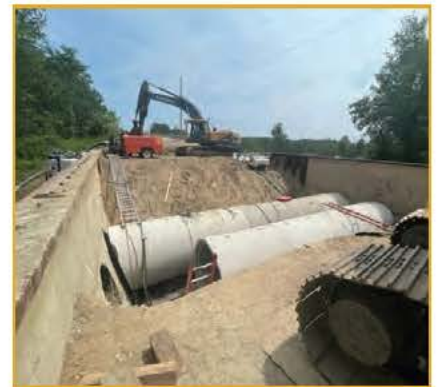
Culvert replacement on Furbush Road
