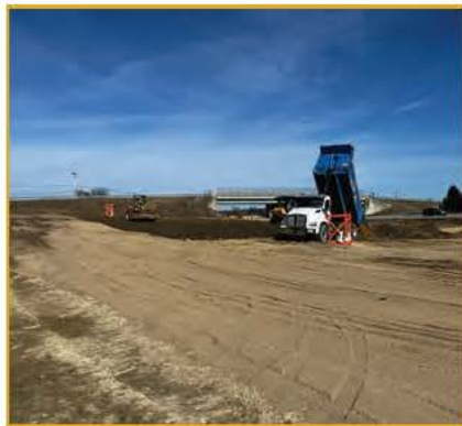
Preloading the southbound ramp area
