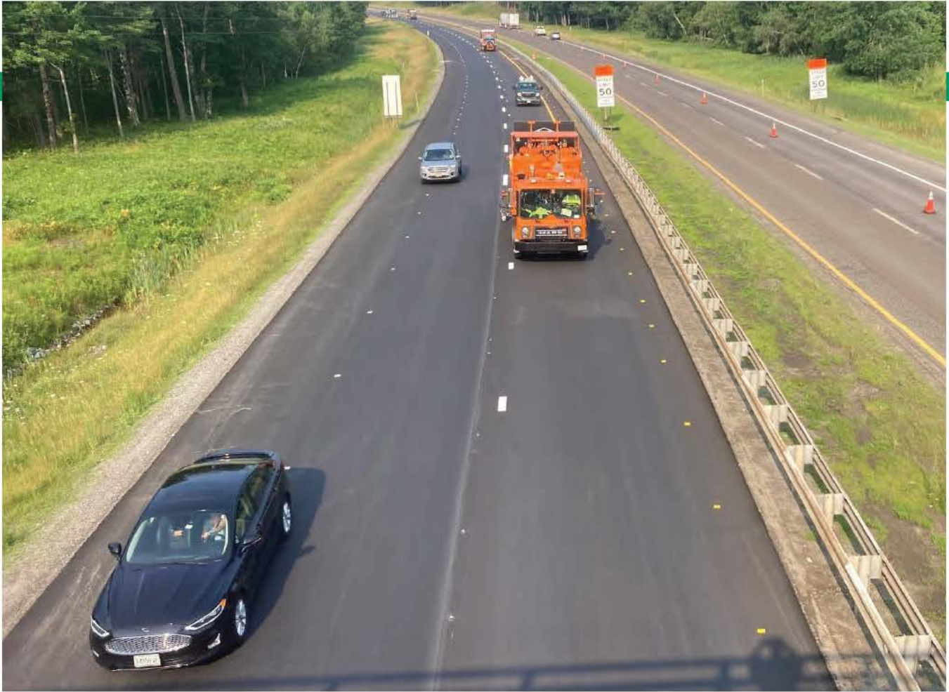
Striping the new pavement Mile 88 to Mile 98, July
