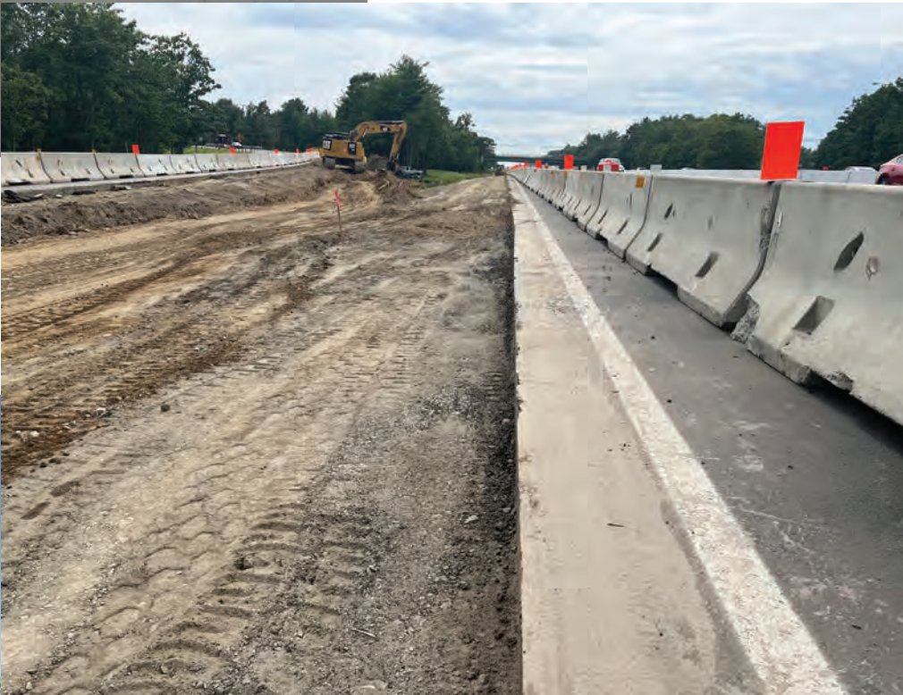
Restoring roadway after toll plaza demolition at Mile 7 in York
