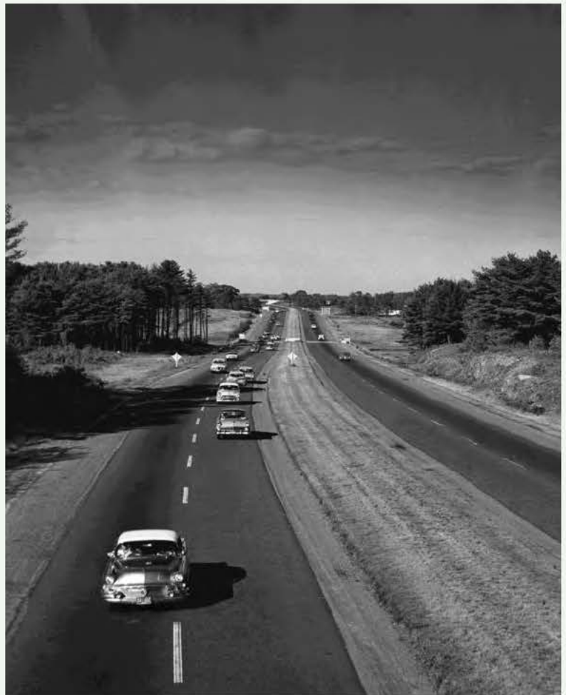
Mile 1 southbound in Kittery. September 3, 1956.
