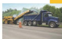
Turnpike contractors recycle pavement to reduce truck trips and costs.
