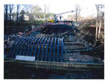
One such example is the Neal Bridge in Pittsfield which was constructed in the fall of 2008. The 27 ft. long arch structure was manufactured from hollow carbon fiber composite tubular arches spaced at approximately 2-feet on center, erected in place and filled with concrete. A corrugated fiber reinforced plastic (FRP) composite decking was installed on top. The head walls were constructed with a FRP sheet pile system.
