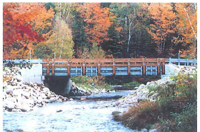
West Branch Bridge, Rt. 17 Byron
