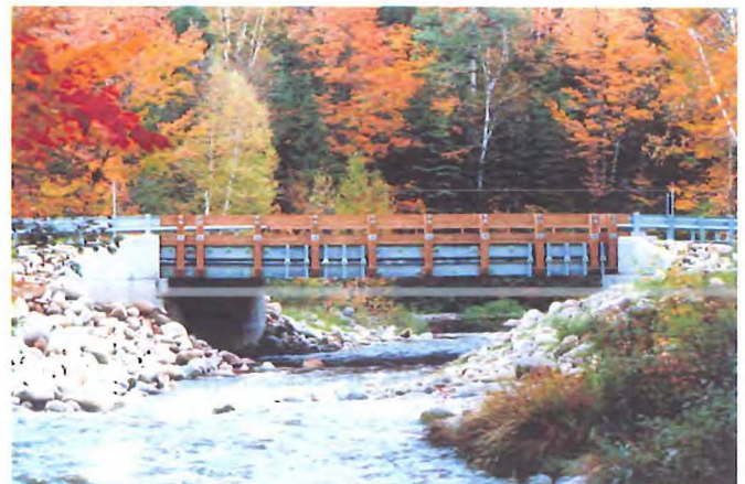
West Branch Bridge, Rt. 17 Byron
