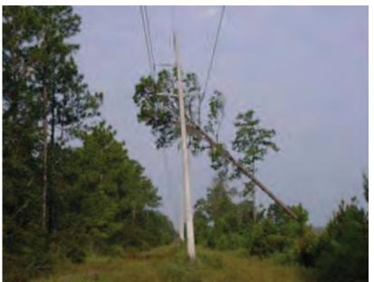
Figure 3-1. Tree falling into transmission lines.
