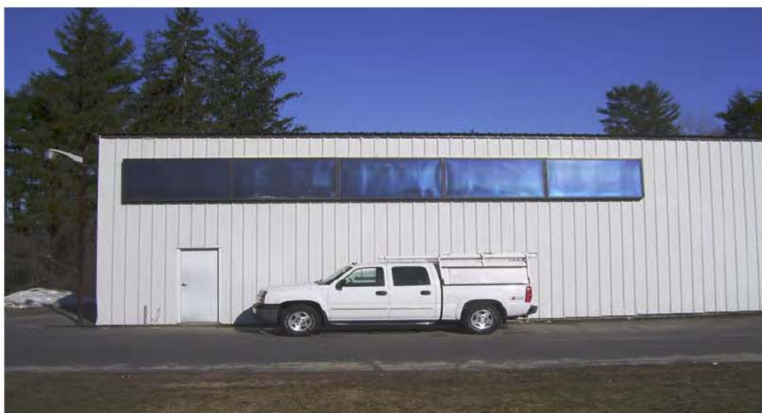
Solar hot air flat plate panels, Gorham. Installed by Jim Robertson of Mainly Plumbing
