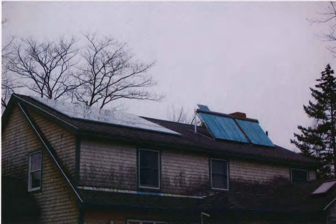
(Solar electric system (2.1 kW) (left) and solar hot water system (right), Brunswick, ME. Installed by Liberty Energy Works LLC.)
