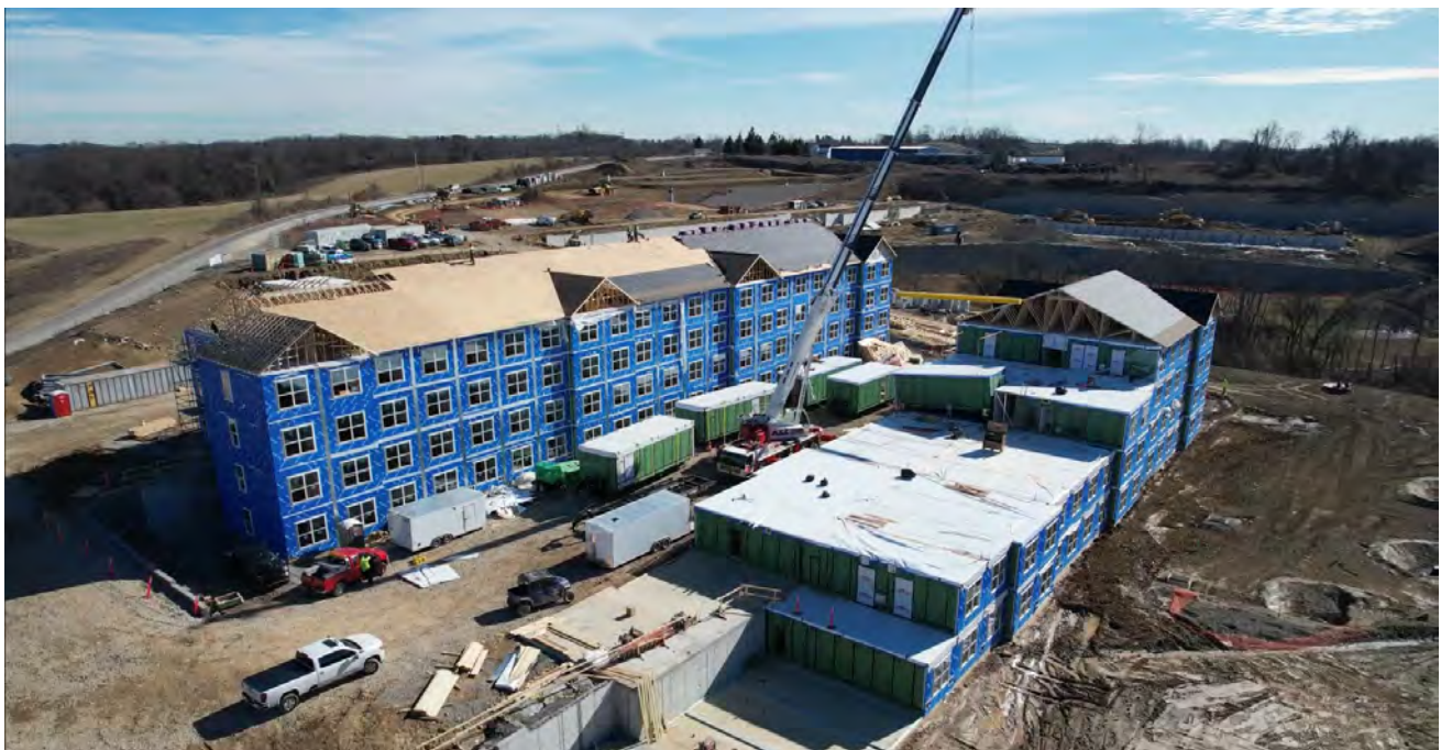
Multifamily modular buildings under construction by Greystar in Elizabethtown, Pennsylvania
