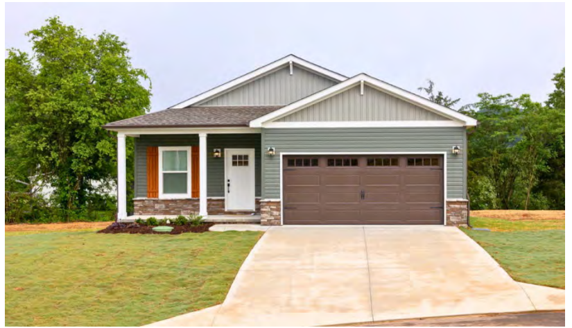
Clayton Homes CrossMod example in Knoxville, Tennessee
