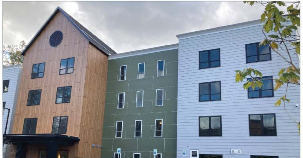
Lewis H. Emery Apartments in Westbrook, 30 new construction units for older adults, funded in part by the State HOME Fund.
