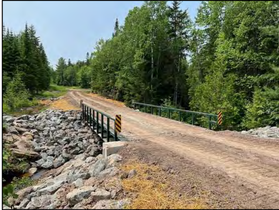
A folding steel temporary bridge installed at the Eagle Lake Unit, BPL Northern Region. The bridge addressed a barrier to fish passage at this stream crossing and improved access to a significant amount of upstream trout habitat.
