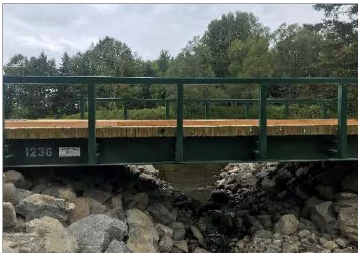
New bridge to enhance stream and riparian area function at Bigelow Unit, BPL Western Region
