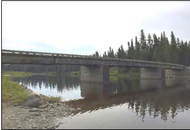
Rehabbed Henderson bridge over the Allagash River, BPL Northern Region
