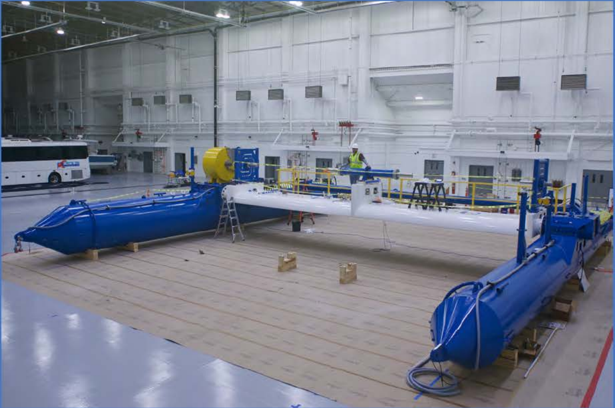
ORPC RivGen Power System being built at Brunswick Landing, Maine (Source ORPC)
