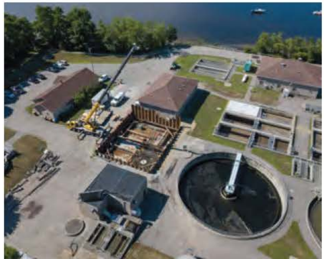
Aerial views show the progress of the $50 million Water Resource Recovery Facility Upgrade project in Saco. The project consists of a new treatment building with aerobic granular sludge treatment processes, secondary filtration, and UV disinfection with upgraded grit removal and solids handling, as well as the conversion of existing clarifiers for additional stormwater storage and site grading alterations to mitigate tidal flooding from the adjacent Saco River.
