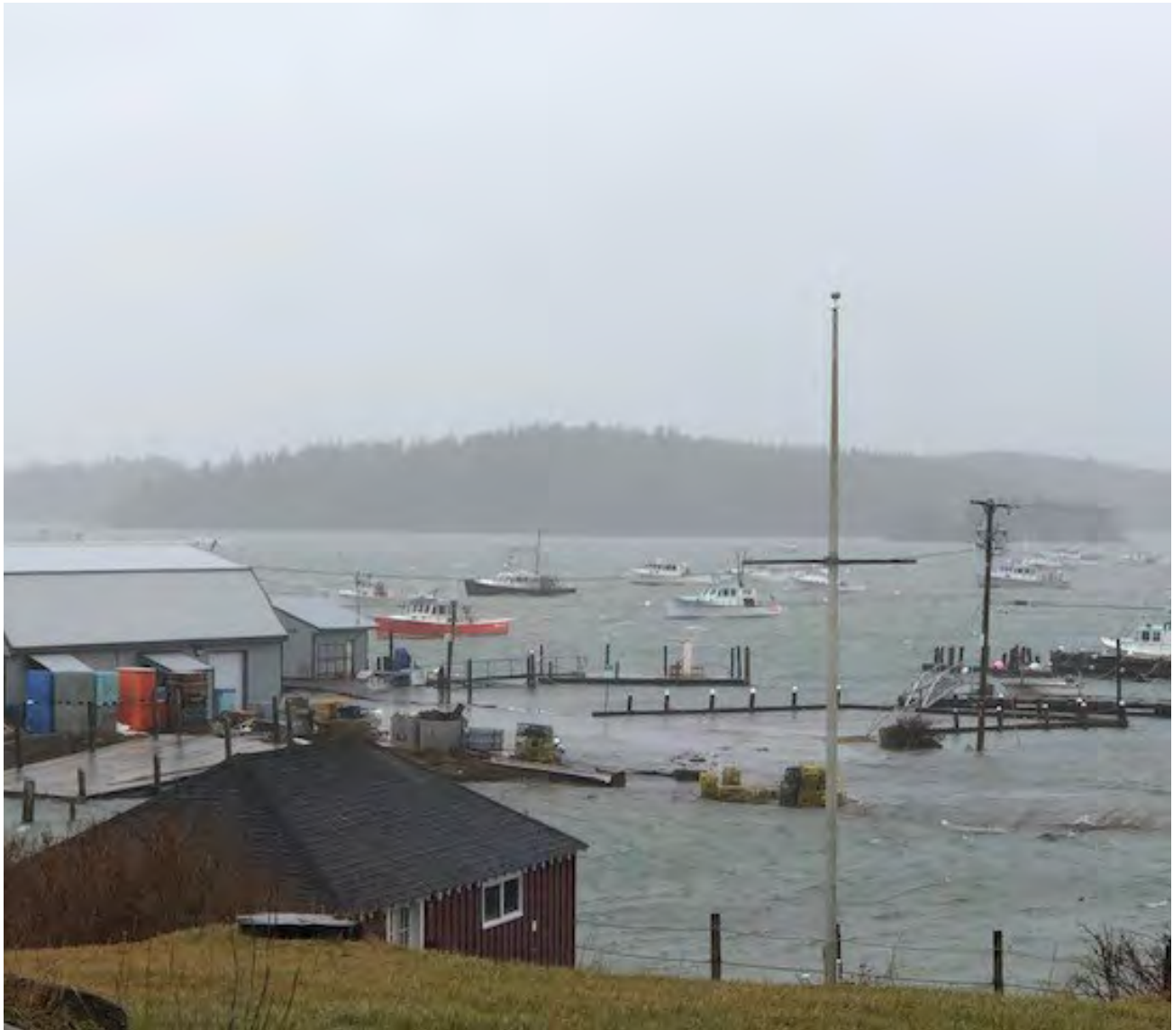
Damaged waterfront structures at the Stonington Co-Op show the force of storm surge on waterfront infrastructure.
