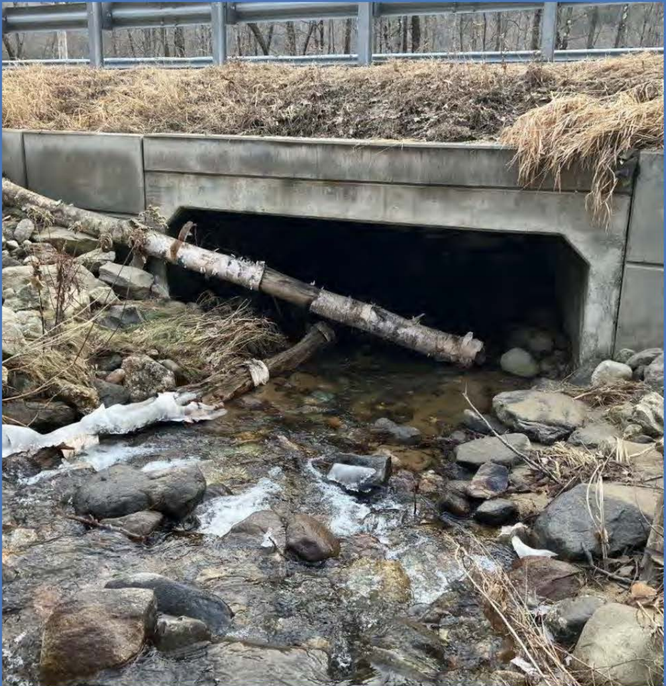
A stream crossing on Route 2 near New Sharon was improved in 2023 and survived the flooding that December. Credit: Maine DOT
