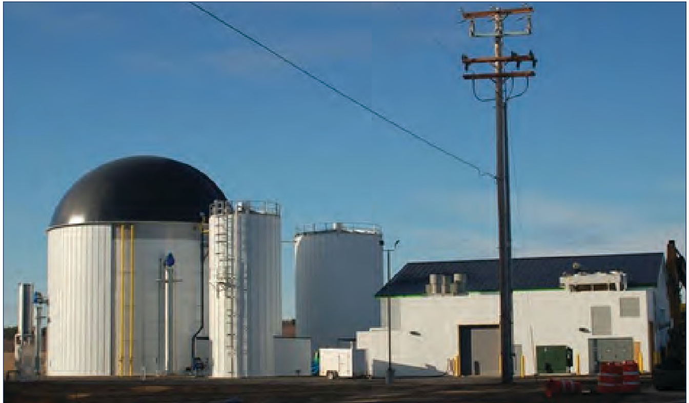
The anaerobic digester is just off the aircraft apron south of Hangar 5 at BXM. The plant can generate up to 1 MW of electricity for Brunswick Landing
