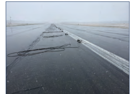
Center line runway lights were removed earlier this year as MRRR works to convert the airport to civilian usage.
