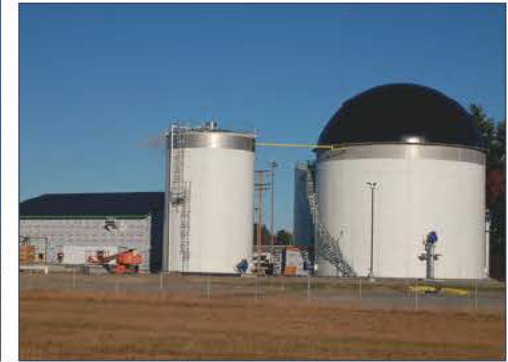
Construction is underway on the renewable energy plant at Brunswick Landing. It is located just off the aircraft apron south of Hangar 5 at Brunswick Executive Airport (top right). Once operational, the plant, which uses an anaerobic digester to produce biogas, will generate up to 1 MW of electricity.
