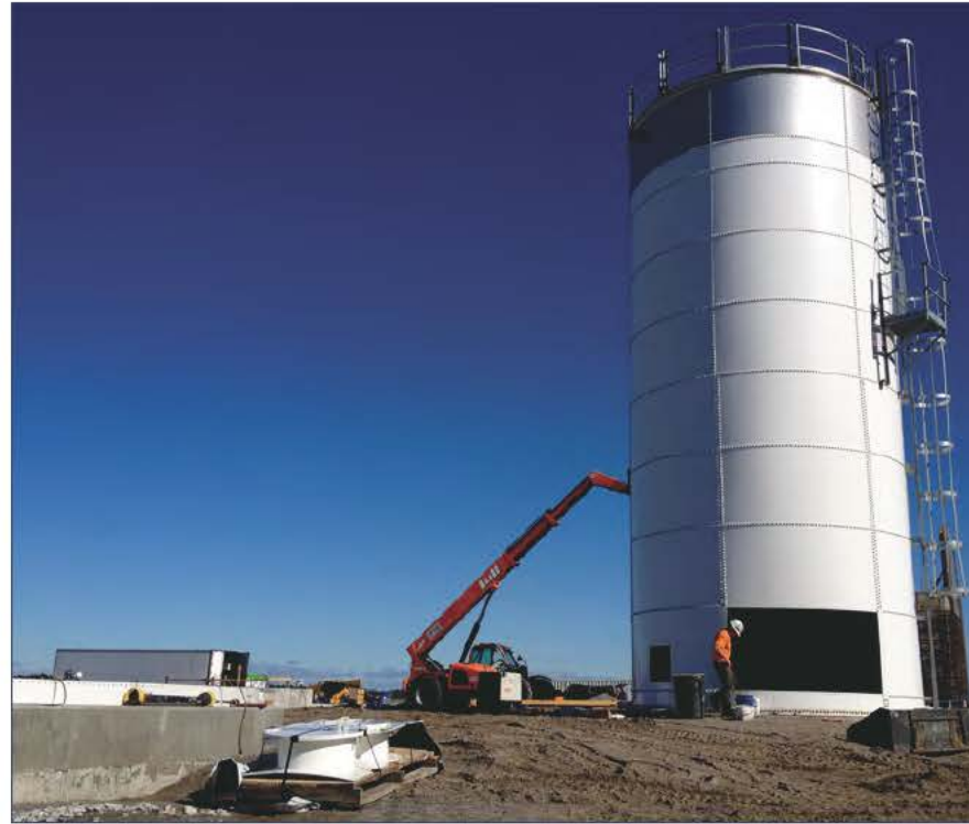
Construction is underway on the renewable energy plant at Brunswick Landing. It is located just off the aircraft apron south of Hangar 5 at Brunswick Executive Airport (top right). Once operational, the plant, which uses an anaerobic digester to produce biogas, will generate up to 1 MW of electricity.
