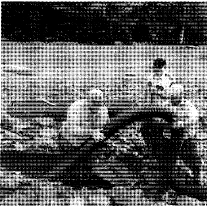
Installing 3 siphon tubes to maintain flows in Martin Stream, Autumn 09
