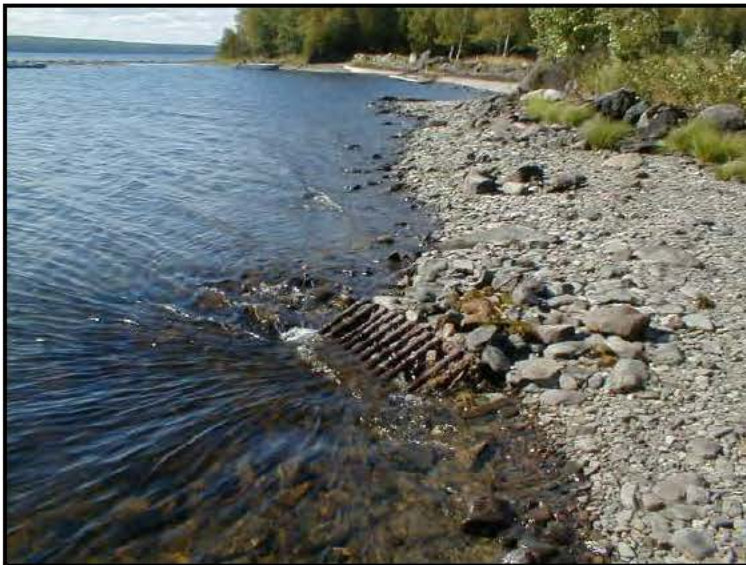
(Left) The Grate and Culvert Enabling Water to Pass through Earthen Lock Dam. Note, photo represents low lake level. (2002 Photo)
