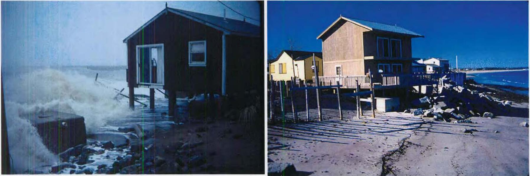
Despite the threat of imminent collapse and a long-term erosion rate of 2 to 3 feet per year, this Saco property was enlarged prior to being destroyed in 1991. MGS File Photos by S. M. Dickson, left 1986 and right, 1990.
