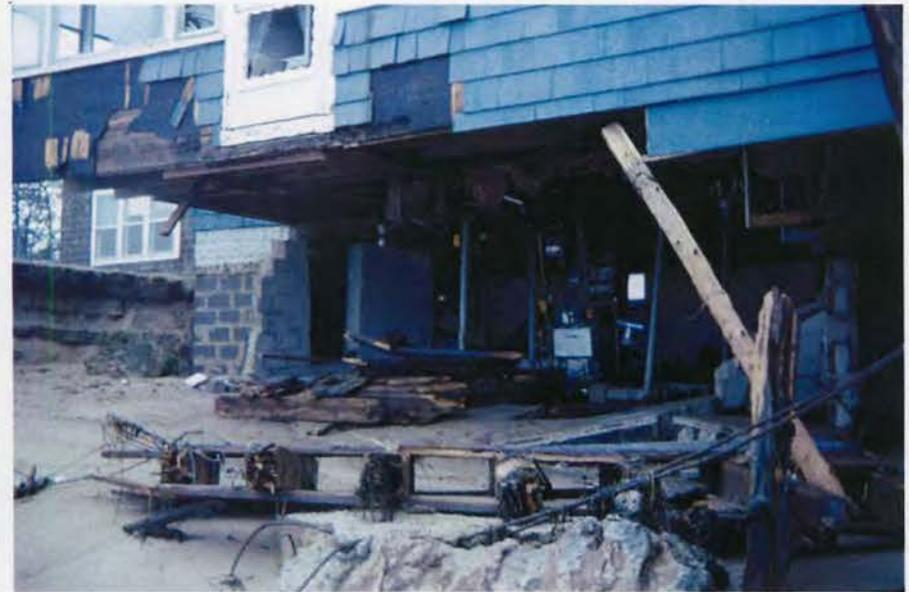
Seawall failure results in rapid release of dune sand and fill from behind the wall. Foundations can be undermined before a storm ends and result in structural damage behind seawalls. MGS File Photos (Wells, 1987 and Saco, 1991) by S. M. Dickson.
