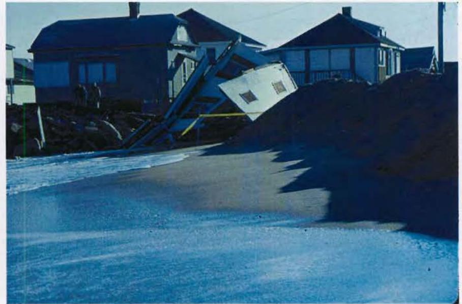
Surf and chronic erosion threaten the Camp Ellis neighborhood. The two homes in the left photo were destroyed by different storms. The house on the left was behind a seawall; the one on the right was not. MGS File Photos by S. M. Dickson, left 1986 and right 1990.
