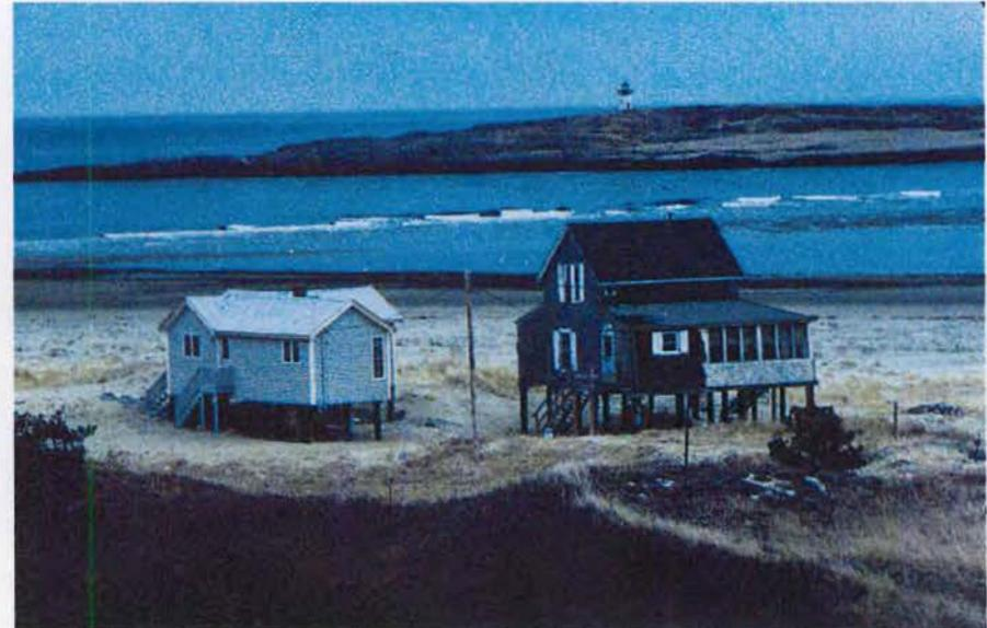
A damaged home at Hunnewell Beach in Phippsburg (left) and the neighboring home were moved landward and raised on posts after erosion in 1983. MGS File Photos by J. T. Kelley, left, 1983 and by S. M. Dickson, right, 1989.
