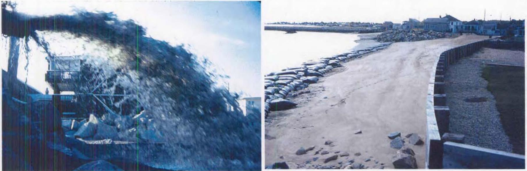
Beach nourishment places additional sand on the beach profile to reduce the sand deficit. Sand bags were placed on the beach to attempt to slow the erosion rate in Saco. MGS File Photos by S. M. Dickson, 1992 left and J. T. Kelley, 1992, right.
