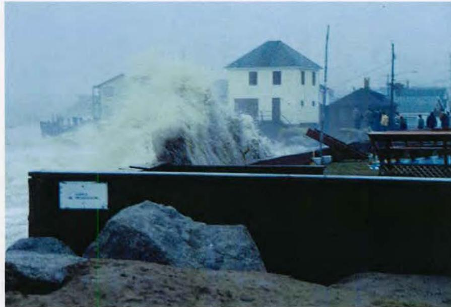
Seawalls result in wave reflection that causes enhanced beach scour in front of the wall. Over time the beach will lower and expose more of the wall. Continued erosion in front of the wall leads to a narrower beach and the need to reinforce or enlarge the wall to increase its resistance to wave action. MGS File Photos (Goose Rocks Beach, Kennebunk, 1990 (left) and Saco, 1986) by S. M. Dickson.
