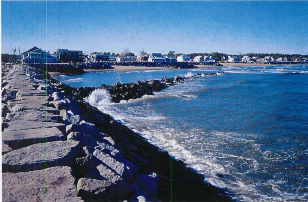
Coastal engineering at tidal inlets alter the natural movement of sand. In Saco, the jetty prevents Saco River sand from reaching the beach and wave reflection causes accelerated beach erosion and longshore drift. There are other federal jetties in Wells, Kennebunk, and Scarborough adjacent to beaches. MGS File Photo by S. M. Dickson, 2002.
