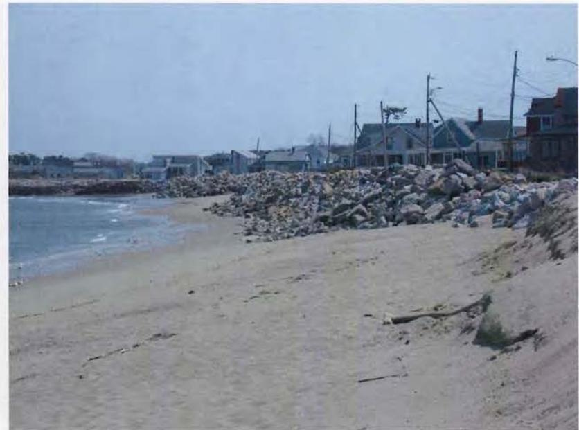
Sheet pile for reinforcement of seawalls along Beach Avenue in Kennebunk. Riprap in Saco slumps on the beach over the upper part of the beach profile. MGS File Photos by S. M. Dickson, 1999, left and 2002, right.
