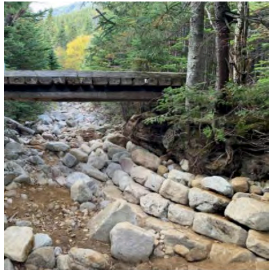
Upper Saddle Brook Bridge and armored streambank
