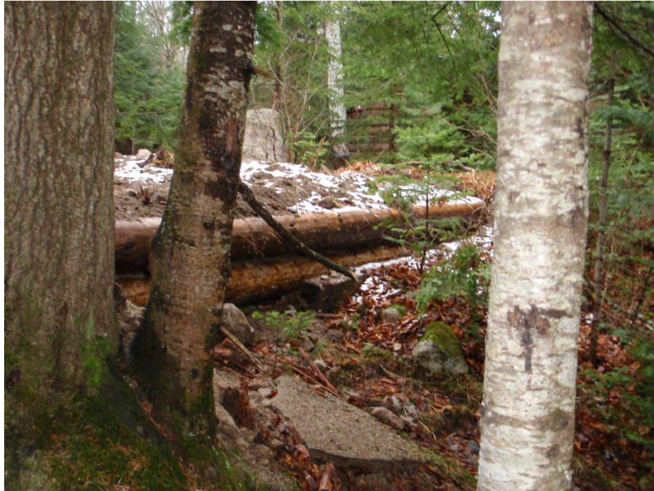
Traditional round log cribbing at Katahdin Stream Campground lean-to nine. Photo courtesy of Stewart Guay
