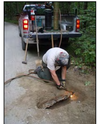
Wayne Brooker removing a culvert in the road.
