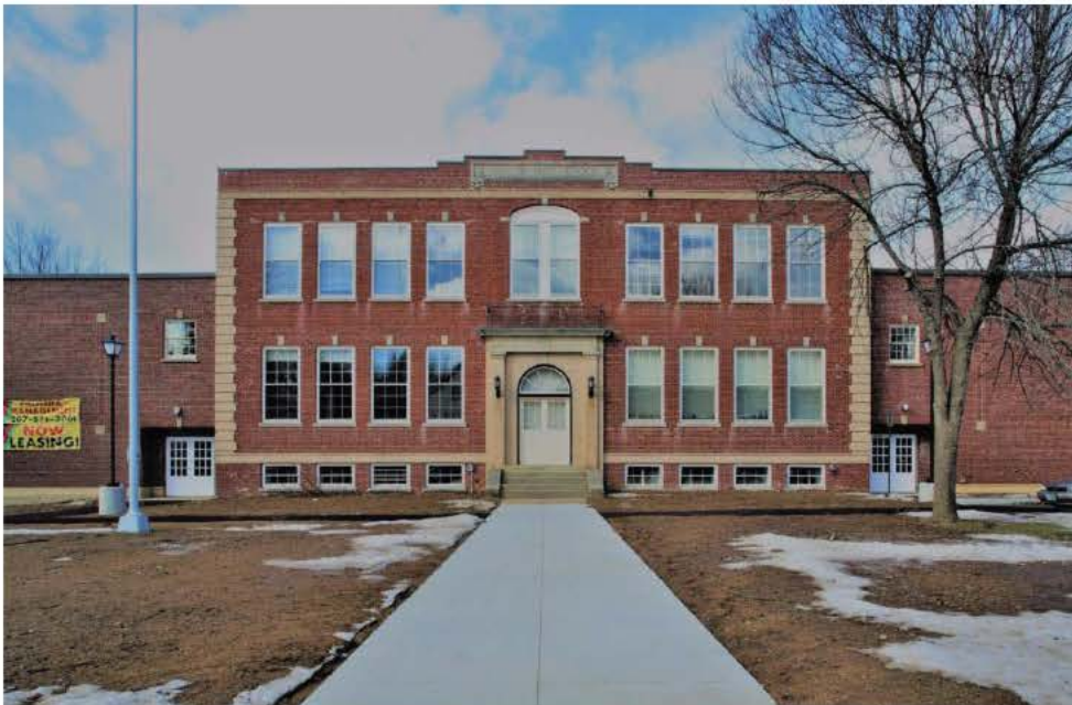
Sullivan School Apartments, Berwick
