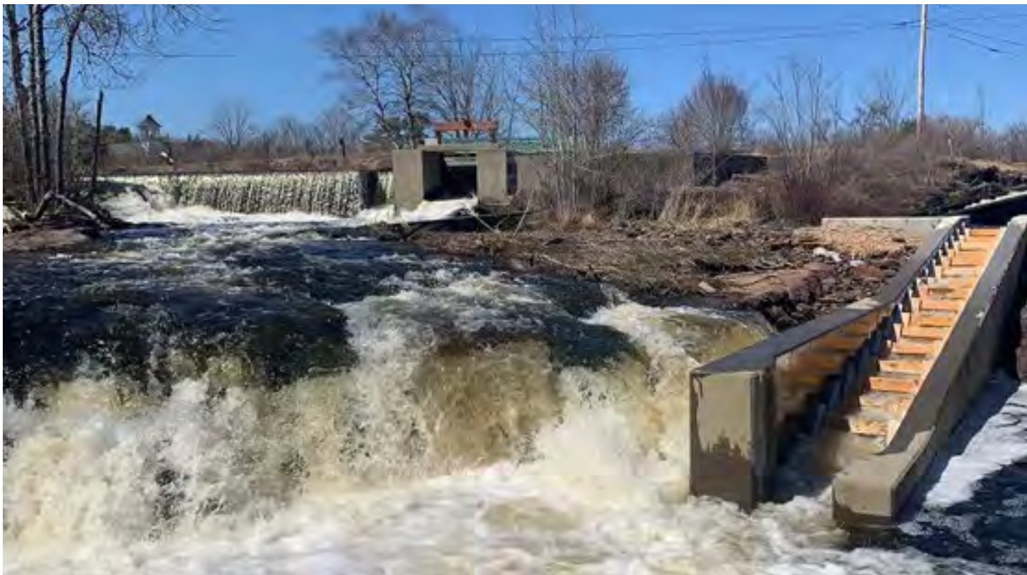
Fish ladder on the Pennamaquan River, Pembroke, Maine. Photo by Chris Johnson.
