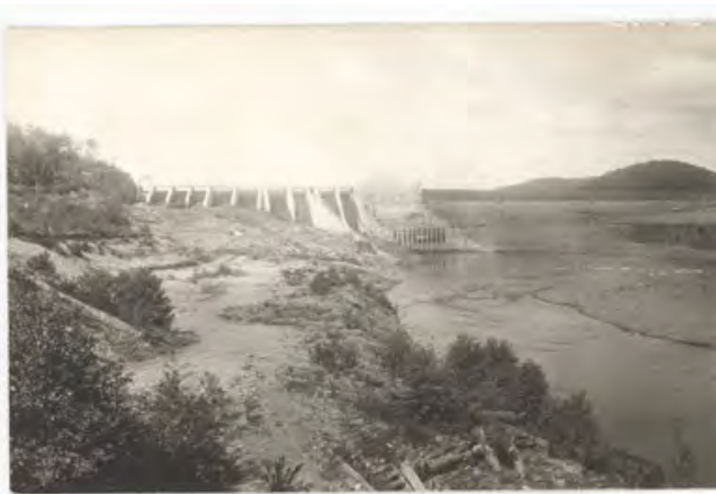
View of Wyman Dam (1928-1931) on the Kennebec River in Moscow, seen looking north. Courtesy of the Maine Historic Preservation Commission, Augusta, Maine.
