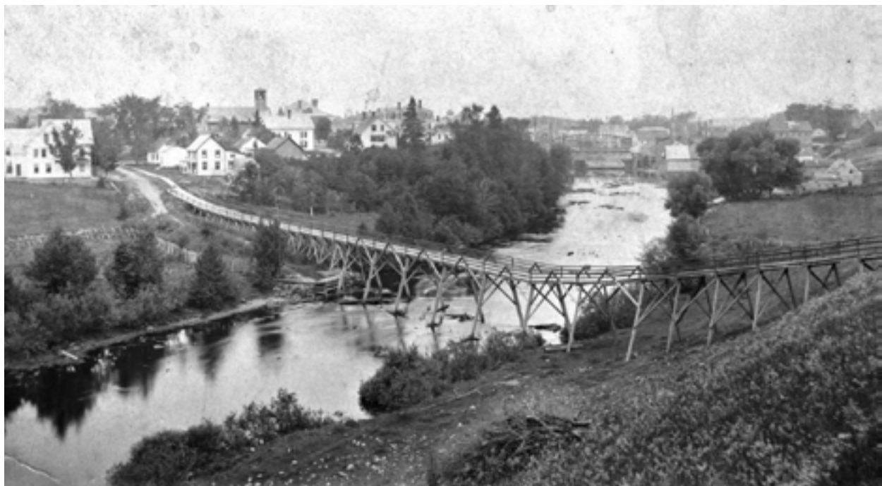
Looking south to lenticular through truss on North Street in distance. Photo by Edward B. White.
