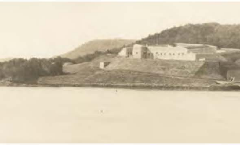
Fort Knox (1844-64, principal architect General Joseph G. Totten) in Prospect, seen from Bucksport across the Penobscot River. Courtesy of the Maine Historic Preservation Commission, Augusta, Maine.
