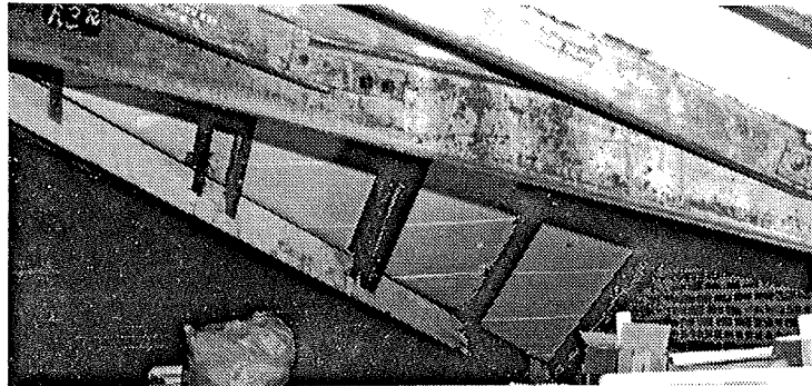
FIG. 12A STEEL ROOF RAFTER SYSTEM SHOWING FIG. 12B GYPSUM PANELS, BRICK AND TILE FIG. 12C WALK. IN 12D NOTE NAILS FROM FIG. 12D ROOFING EXTENDING THROUGH GYPSUM
