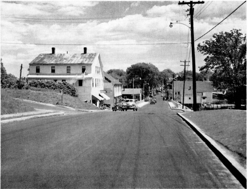
Damariscotta-Newcastle, U. S. Route No. 1
