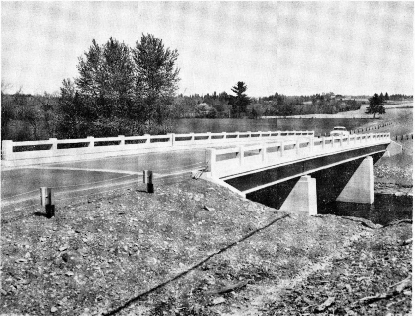
Caribou, Little Madawaska River Bridge
