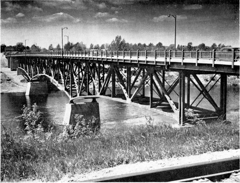
Caribou, Aroostook River Bridge
