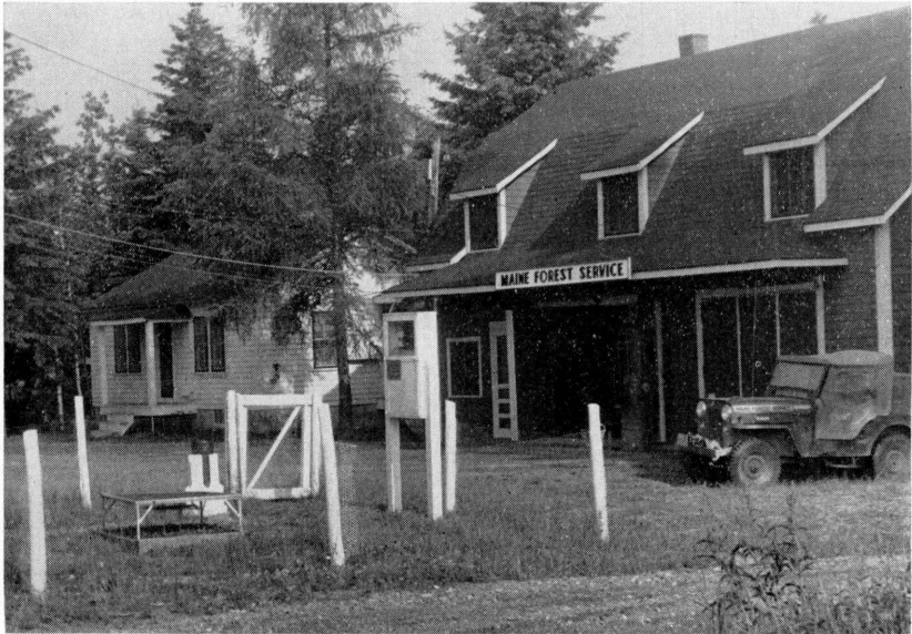
Warden Unit Headquarters
