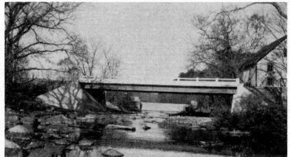
HEAD TIDE BRIDGE ALNA
