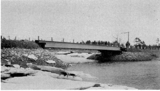
LOWER ABAGADASSETT BRIDGE BOWDOINHAM
