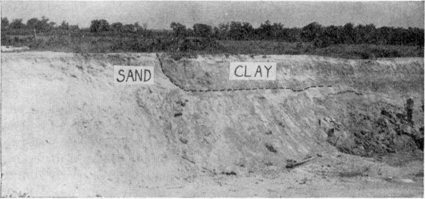
**Figure 1.** Sandpit near Cash Corner, S. Portland. Clay overlying sand (contact marked by broken line).
