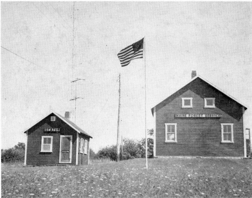
WINDSOR HILL RADIO RELAY STATION
