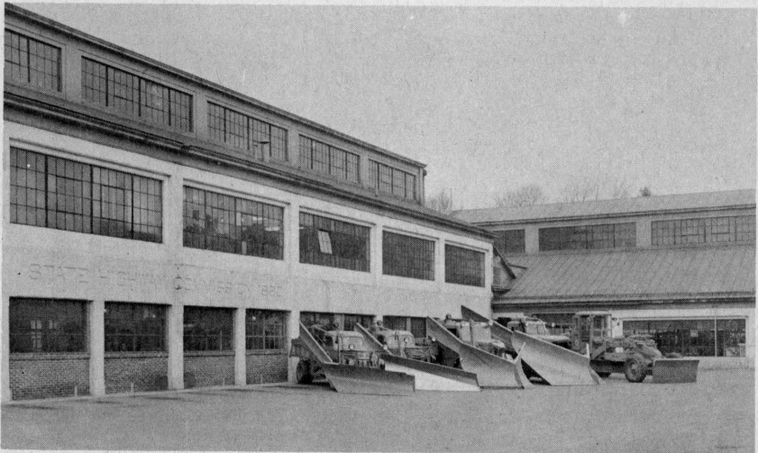
STATE HIGHWAY GARAGE
