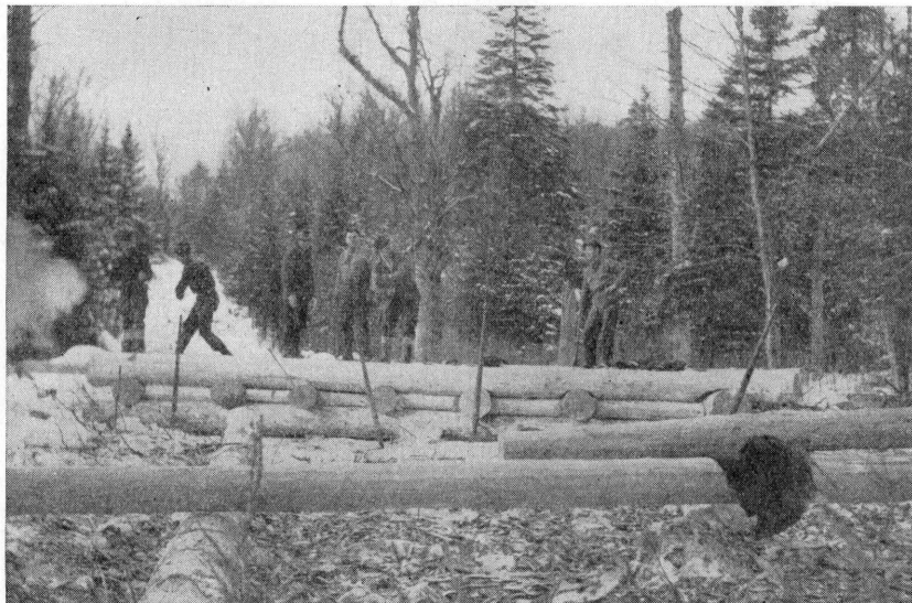
Log culvert under construction from Greenville Camp
