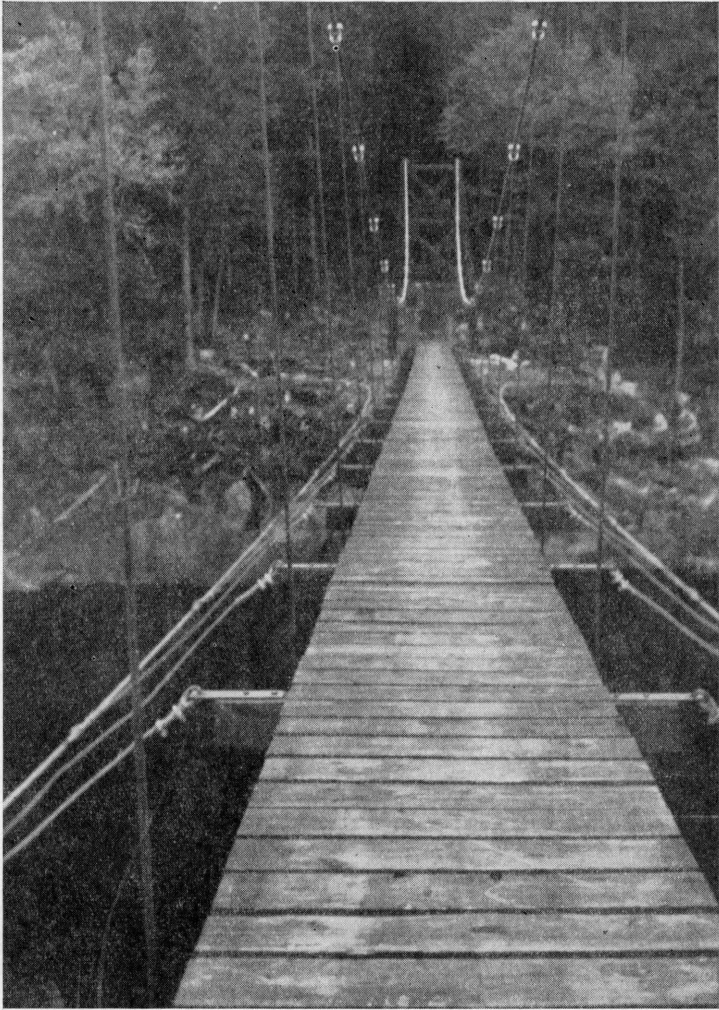
Sourdnhunk Suspension Foot Bridge
