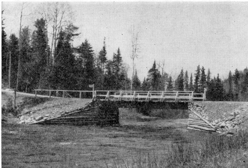
Grand Lake Truck Trail, Seboeis Bridge: Wooden abutments, steel girders
