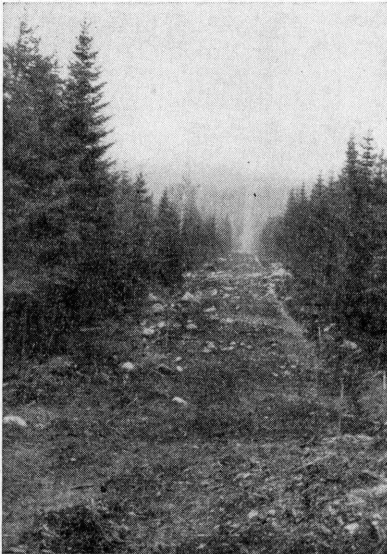
Grubbed right of way on Truck Trail from Rangeley to Wilson's Mills
