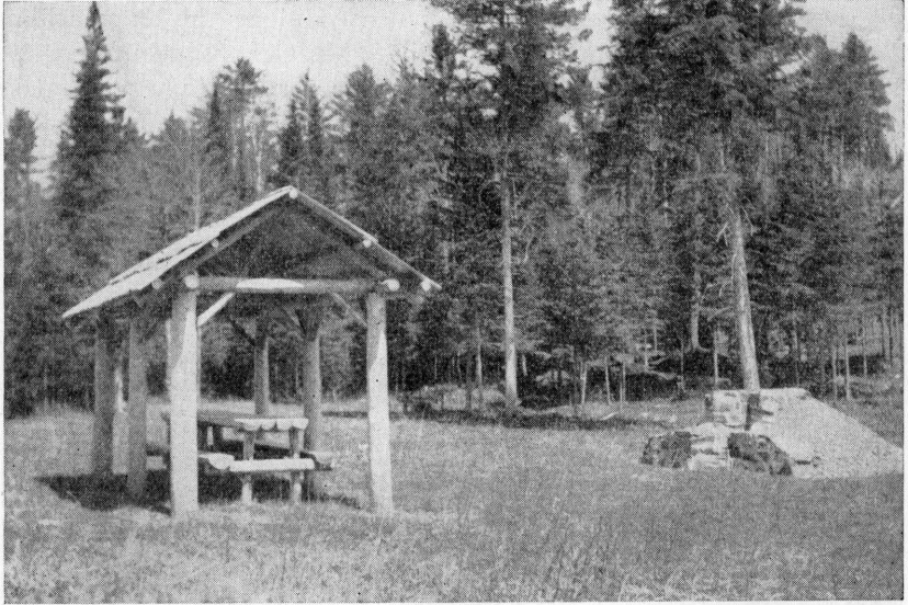
Luncheon shelter built of local materials, with split roof and fireplace: at Seboeis Stream
