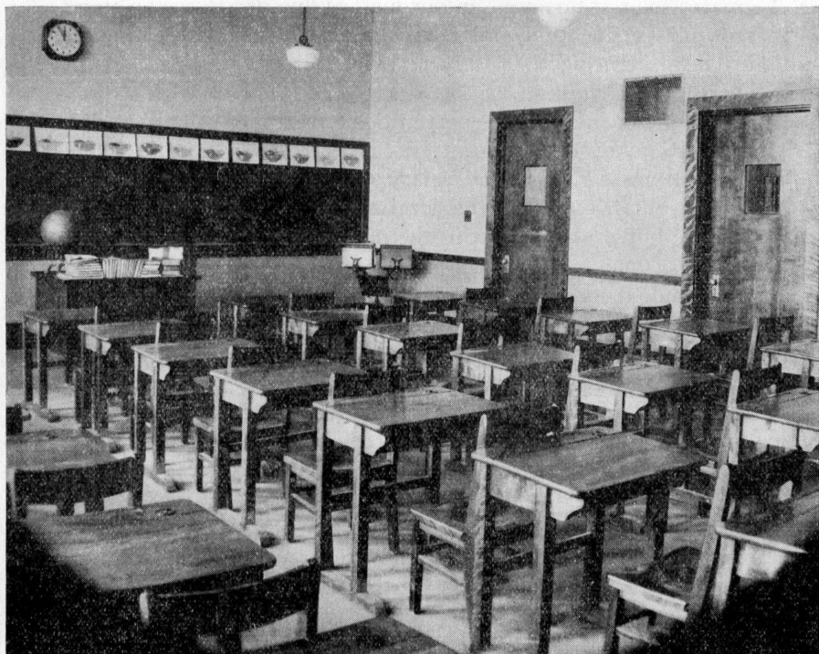
Interior View of Hawthorne Two-room Rural School Building, South Sanford, Maine
