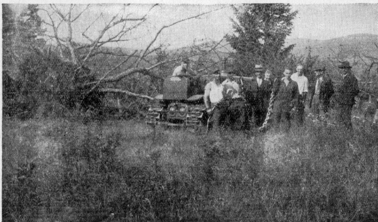
Equipment and Crew Used in Removal of Trees
