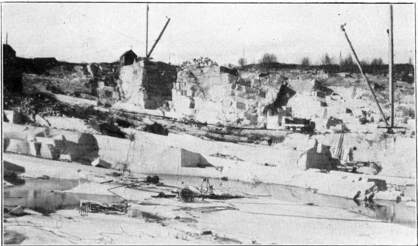
Figure 3-B. Sheet Structure in North Wall of Lithgow Hill Quarry Notice parallelism of sheet structure with the surface and increase in thickness of the sheets downward.
