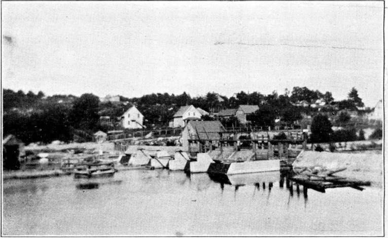
FISH SCREEN AT GRAND LAKE STREAM, WASHINGTON COUNTY
