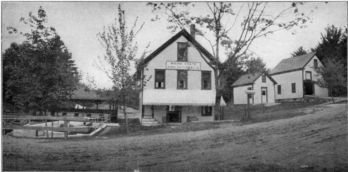
STATE FISH HATCHERY AT CAMDEN, KNOX COUNTY.
