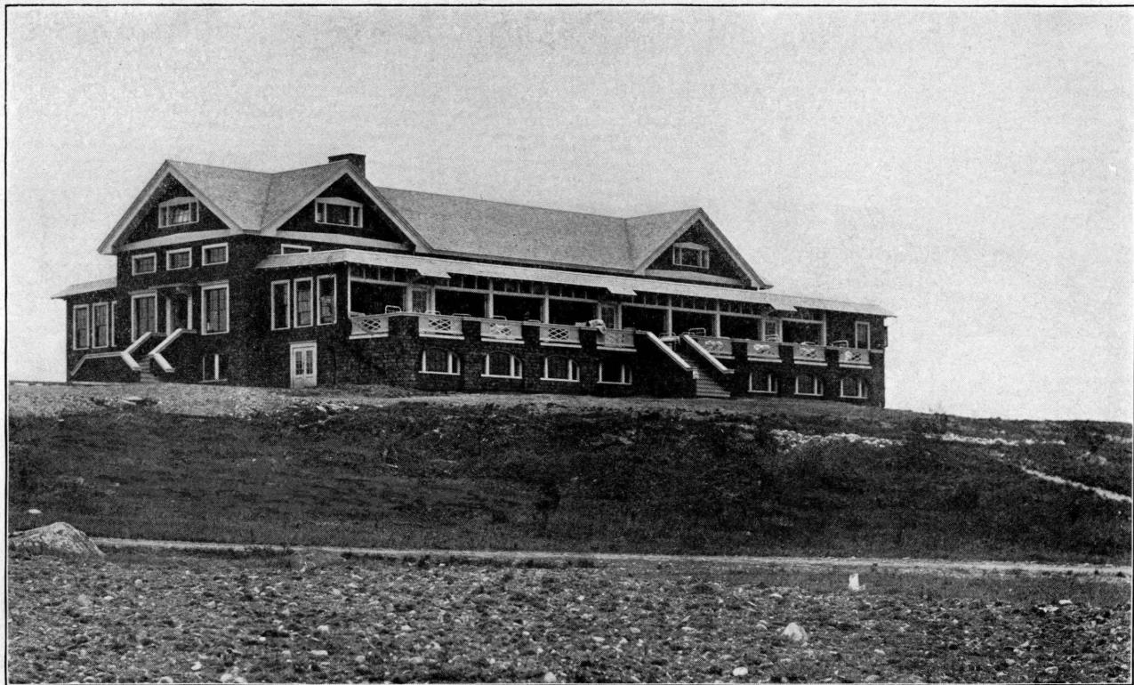
Central Maine Sanatorium—Chase Memorial Building.
