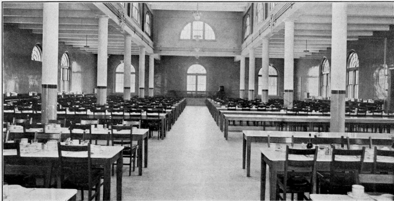
Congregate Dining Room, Bangor State Hospital, Bangor, Maine.
