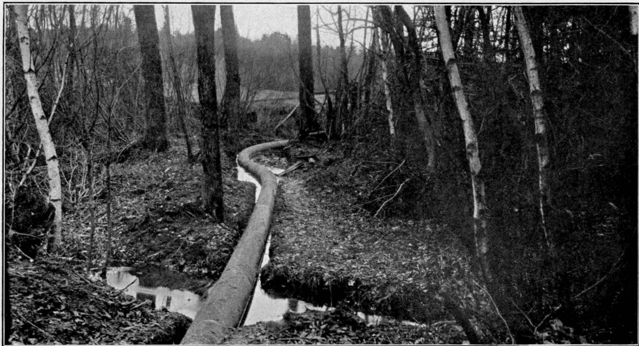
Wood Pipe Line at Monmouth Hatchery.
