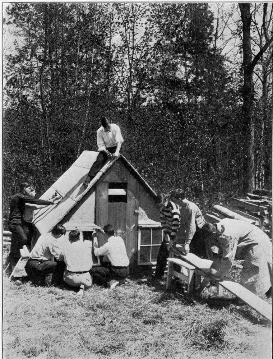
Poultry House Construction at Parsonsfield Seminary.
