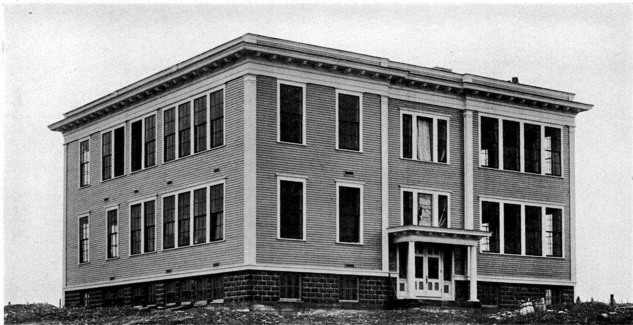
High School and Grade Building, Limestone, Erected 1913.
