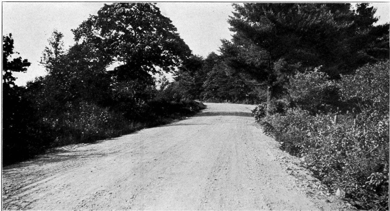
Section of Gravel Road in Kennebunkport.
