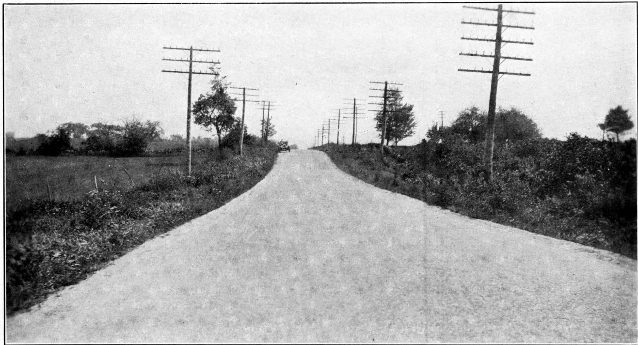
Bituminous Macadam—Kittery-York Section.
