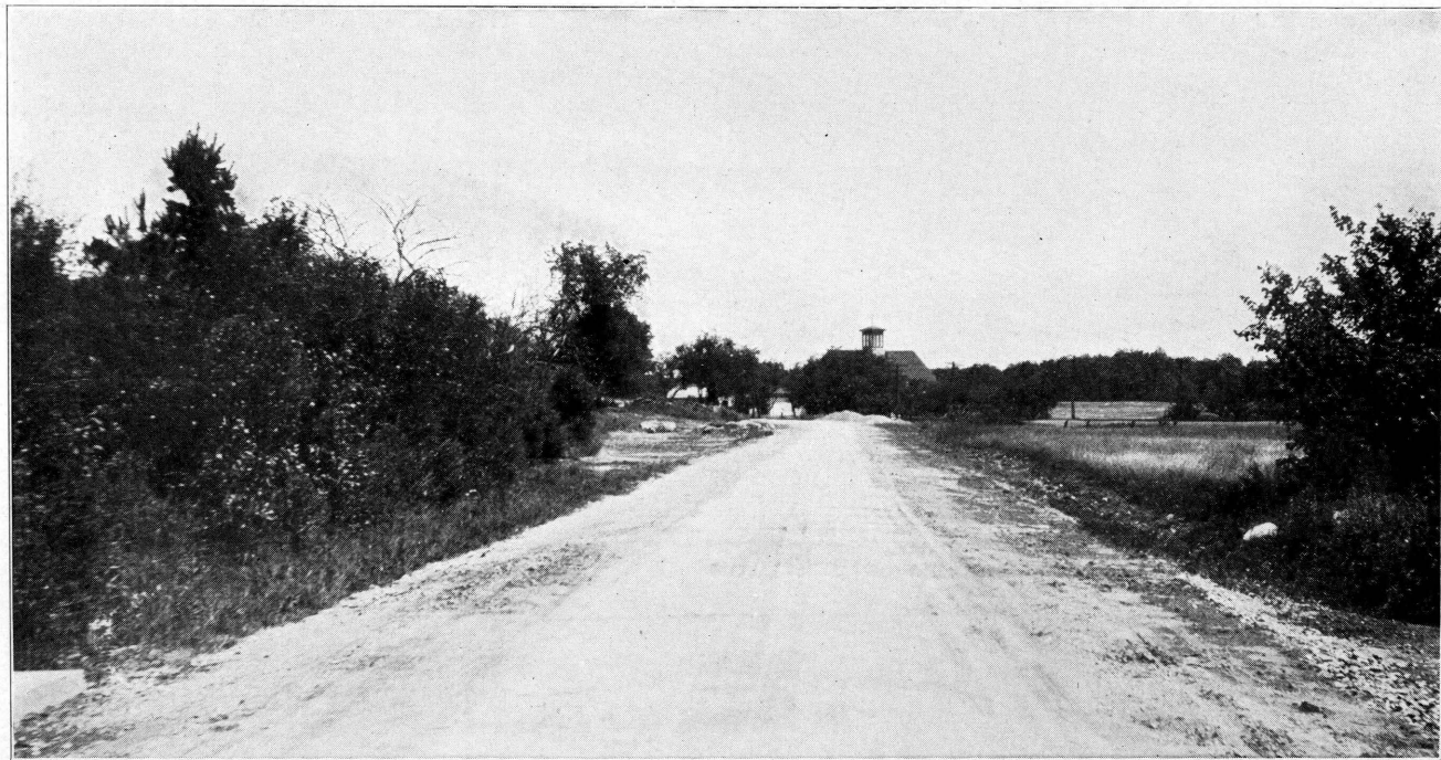
No. 3. Concrete—Kennebunkport Section.
