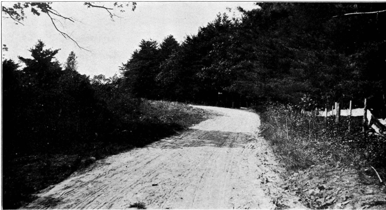
Section of State Aid road in Kennebunkport before improvement.
